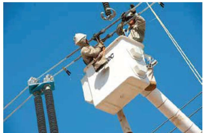
dures was the ability to adapt to job irregularities. A necessary adaptation that occurred early in the project was related to the bundled conductor, which sat in a vertical configuration rather than the tradition horizontal configuration. To most efficiently tackle this issue the team needed to adapt both the equipment and the procedures. This first test proved to be a calling card for the entire project as procedures were continually updated to make the project safer and more efficient.
