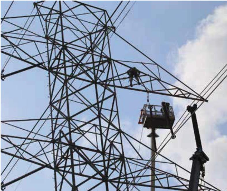
bonded to the conductor, putting them at the same potential as the energized conductor allowing them to physically touch the energized conductor and equipment. To support conductors while unclipping or clipping, the LineMaster Single Point Lifter robotic arm was used. This tool provided safe, secure and controlled support of the energized conductors.
